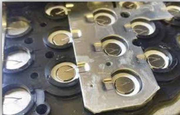
Cells Electrical connection to Bus Bar.
