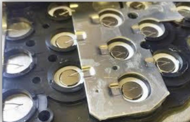
Cells Electrical connection to Bus Bar.
